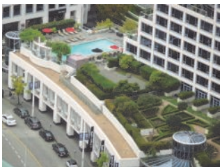
A relatively common sight in Vancouver— gardens on roof tops.
